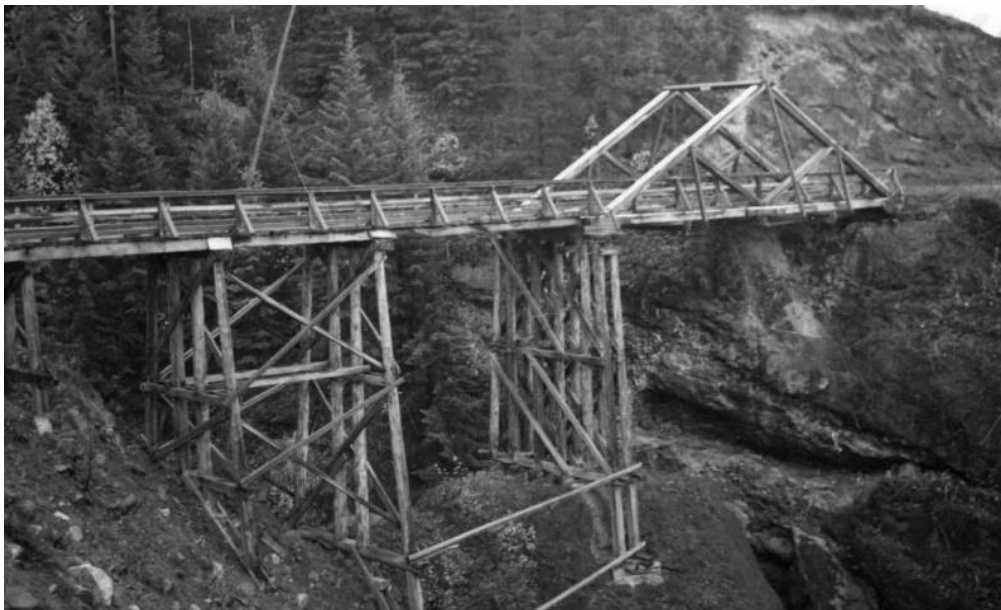
One-way wooden bridge built in 1953, was an improvement over what was originally there (no picture). This is at the 2nd Canyon on the way into the Upper Clearwater area and had an approach of very sharp turns.
